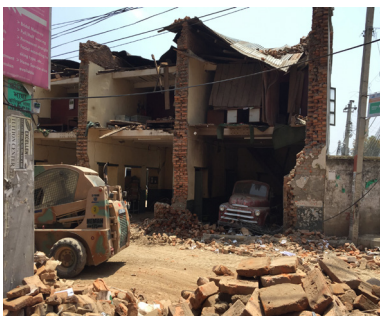
Figure 1 - The front of the antique car museum building fell off completely
